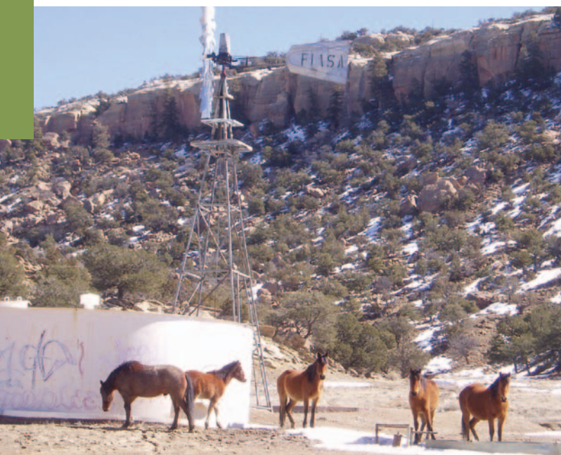
Windmill pumps groundwater into a storage tank on the Navajo Nation.
