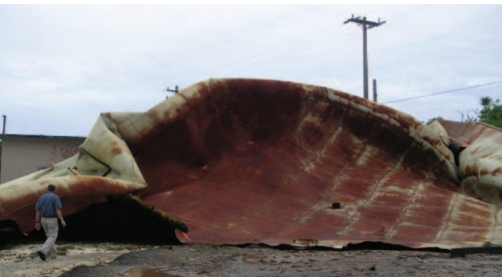
An aging water tank on Saipan that collapsed.
