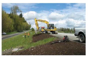
Figure 21. Construction of I-5 Pilchuck vegetated filter strips. Photo illustrates installation of compost amended vegetated filter strips (CAVFS) and modified vegetated filter strips (VFS). (Photo provided by Fred Bergdolt, WSDOT.)
