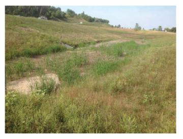
*Figure 19. Sedimentation in floor of Pine Bend infiltration basin after construction.*
