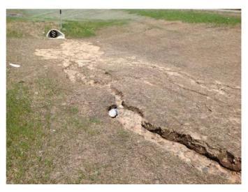
Figure 18. Erosion of side slopes and basin floor in Pine Bend infiltration basin.
