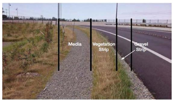
Figure 3. Components of a media filter drain.
