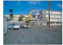
demolishing and downsizing more than 250 buildings (2 million square feet) existing on Johnston Island. Parsons also sorted, transported, placed, and backfilled over all demolition debris on the island and staged recyclable materials for off-island transport.
