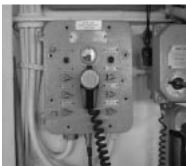
PCB leaks were also found in the remote microphone control station, located in the ship's bridge.
