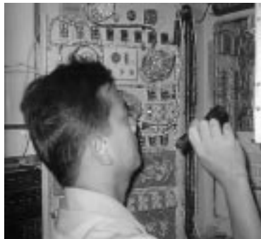
An NEPMU-5 IHO, examines the amplifier oscillator in the IC room of an LPD for PCB leaks.
